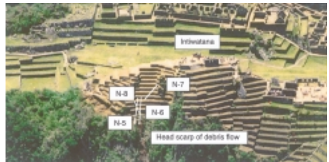
Fig.10 Location of the four sets of simplified type extensometers (N-5,6,7 & 8) installed in the Back Slope beneath the Intiwatana at risk of retrogressing landslide.
