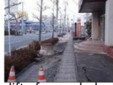
Uplift of a manhole due to liquefaction
