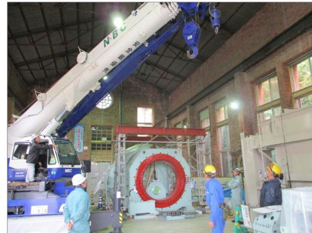
Renovation Project of Ikari Power Station
