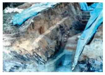
Fig.4. The landslide observed along the trench in 2000. The landslide mass (secondary slide) fell into the inner moat. The base of the mound (the slip surface of the main block) is inclined at 1-3 degrees towards the centre of the mound as a result of the ground subsidence in alluvial clayey deposits under the excess load of the mound. (Photo by Dr. Sangawa)
